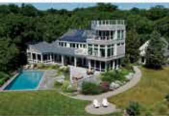
Guilford, Chaffinch Island Road
